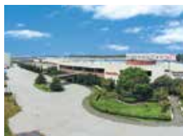
CHINA China Plant (MCC)
